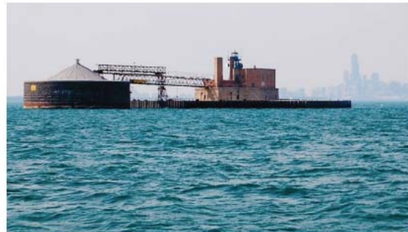
One of Chicago's water cribs, where water is pumped from Lake Michigan to supply parts of our region with drinking water. Photo Credit Eric Allen Roggen
